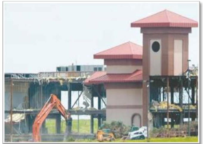
Geneva Lakes Kennel Club demolition, 2014
